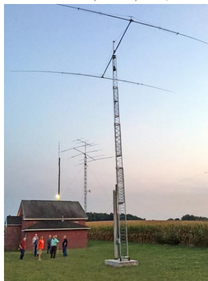
How's this for a sizable beam? This is the Hilltoppers new 40 Meter beam at their clubsite in Red Lion. It is a monster! It sits atop a 70 foot crank up tower. In the background is the club house with a smaller 50 foot tower with a tri-band beam and a 6 meter Yagi. This was taken last Tuesday at a normal monthly meeting of the Hilltoppers Transmitting Association.
