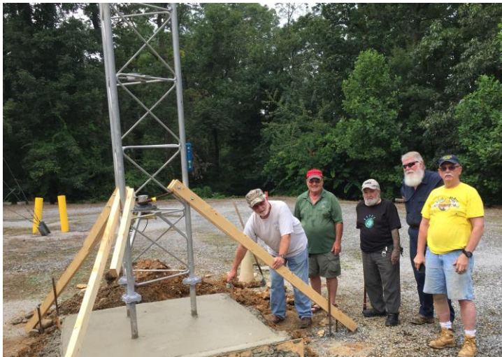
On Monday, July 24th, all of our work culminated in the concrete pour. It took approximately 4.5 cubic yards of concrete to secure the dish supporting structure in place. This was the result of a lot of work by many of our club members!
