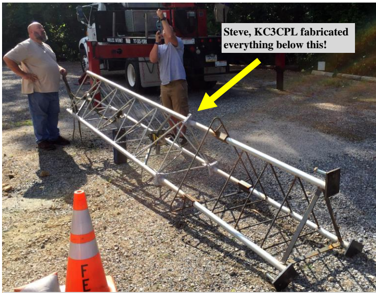
Steve literally fabricated a 6 foot tower extension using stainless steel tubing and rebar. He welded plates on the top that exactly mated with the mounting plates on the bottom of the Rohn tower. On the bottom of his extension, he welded support plates that would sit on concrete blocks in the foundation excavation. On each of these plate was an adjustment bolt, installed through a threaded hole that would be used to perfectly level the tower.
