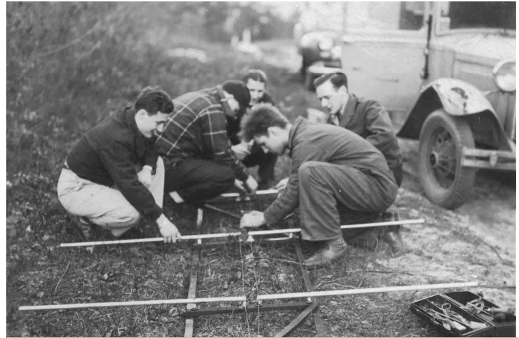
John, W3SST in the front working on what was probably a 2 meter collinear array ... looks like this was taken in the late 1940's or early 50's. This was a REAL homebrew antenna! Check out the car on the right.
