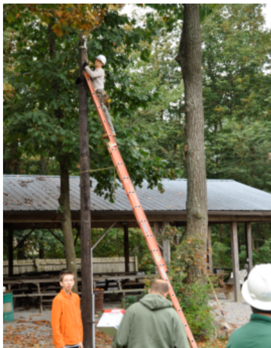
Tim, Dan, and Greg were not the only ones working at height at the Saturday work party. Cameron Bailey, KT3A was up a good 20+ feet installing the new dusk to dawn light.
