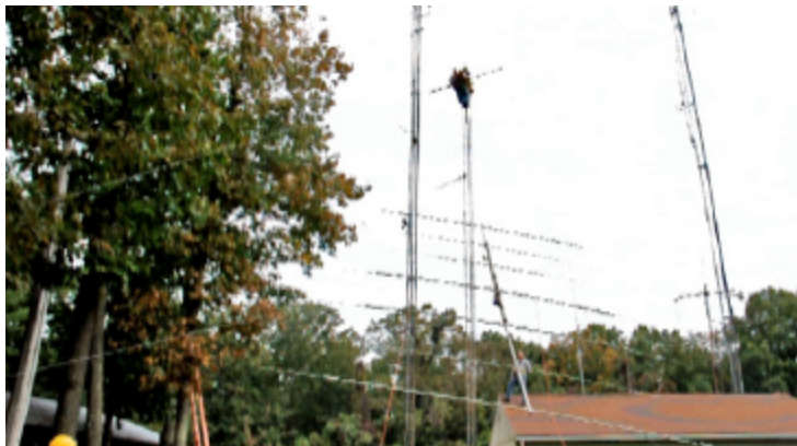
Greg, KE3CW heads up the tower to help Tim, W3TWB guide the TH-7 in place once it is pulled to the top. Dan, N3EEI climbed down to the club house roof where he would remain in case something got hung up on the tower or guy lines. At this point everything looked good. The antenna support ropes were tensioned and the line to actually pull the antenna up attached.
