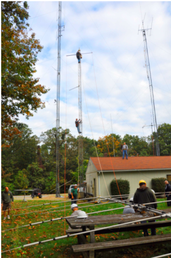
Greg, KE3CW heads up the tower to help Tim, W3TWB guide the TH-7 in place once it is pulled to the top. Dan, N3EEI climbed down to the club house roof where he would remain in case something got hung up on the tower or guy lines. At this point everything looked good. The antenna support ropes were tensioned and the line to actually pull the antenna up attached.
