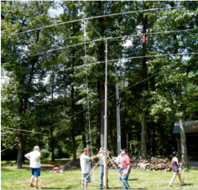
The gang erecting the triband beam provided by the Hilltoppers Club on Saturday morning.
