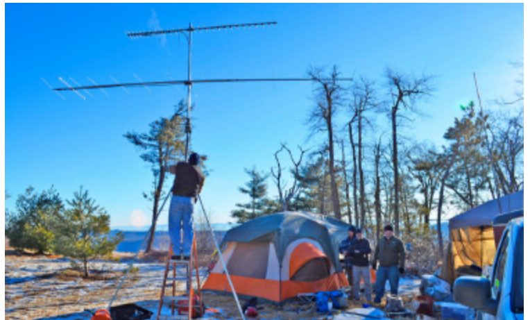
Erecting the 2 meter & 70 CM antenna supports along with the respective antennas went quite well..
